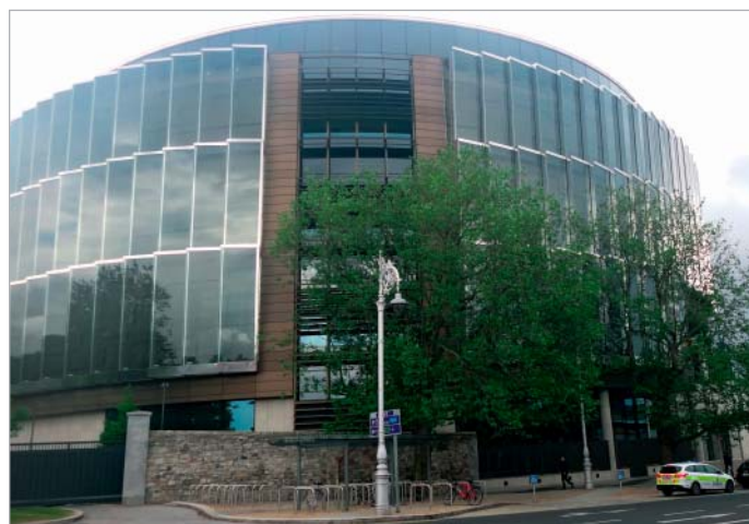
Dublin – budova trestního soudu v Dublinu (The Criminal Courts of Justice)
